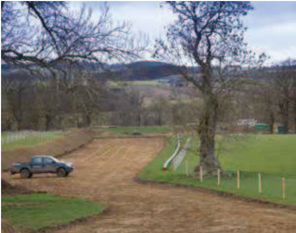
1. Topsoil Strip and Store
