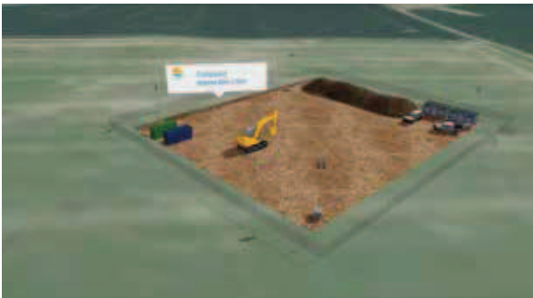
1. Site establishment including topsoil strip and store
