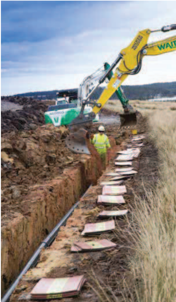
3. Ducts Covered and Protective Marker Tiles Laid
