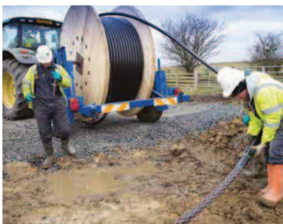
7. Pull cables into ducts
