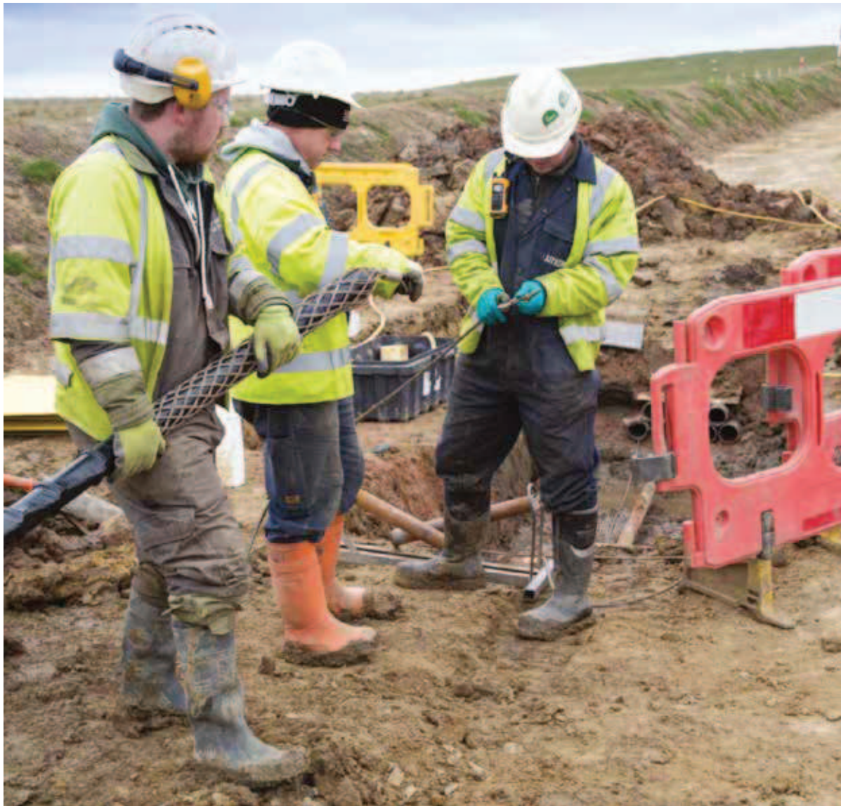
Cable pulling preparation
